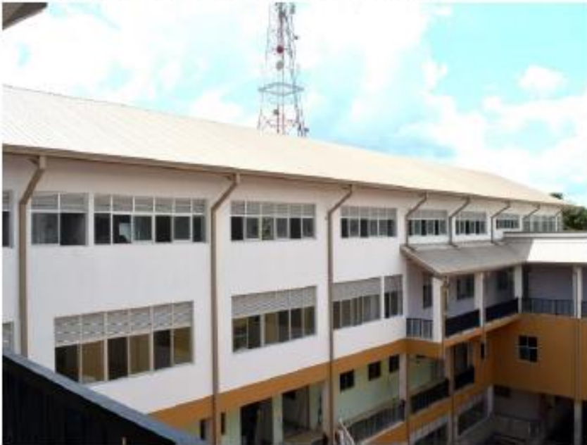
External Finishing Work is Nearly in Completion
