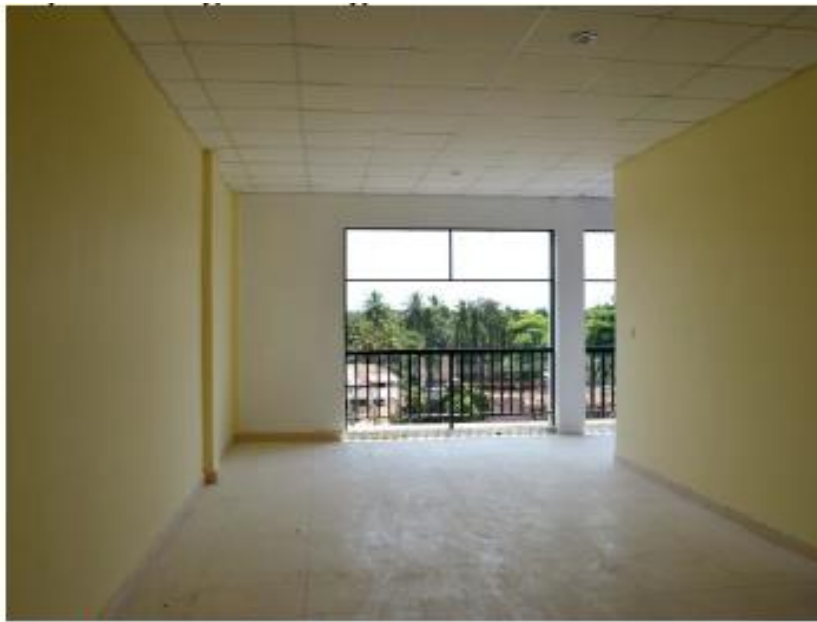
Top Floor Wall and Ceiling Work
