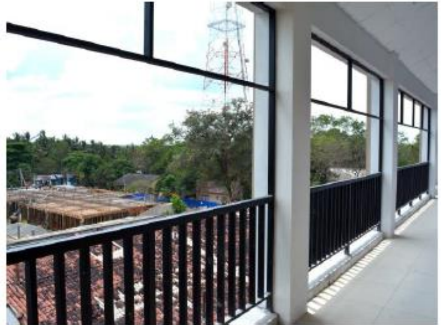
Hand Rail Work Completed
