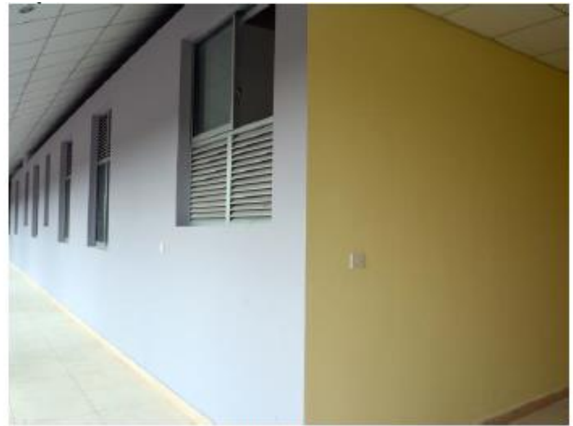
Top Floor Windows
