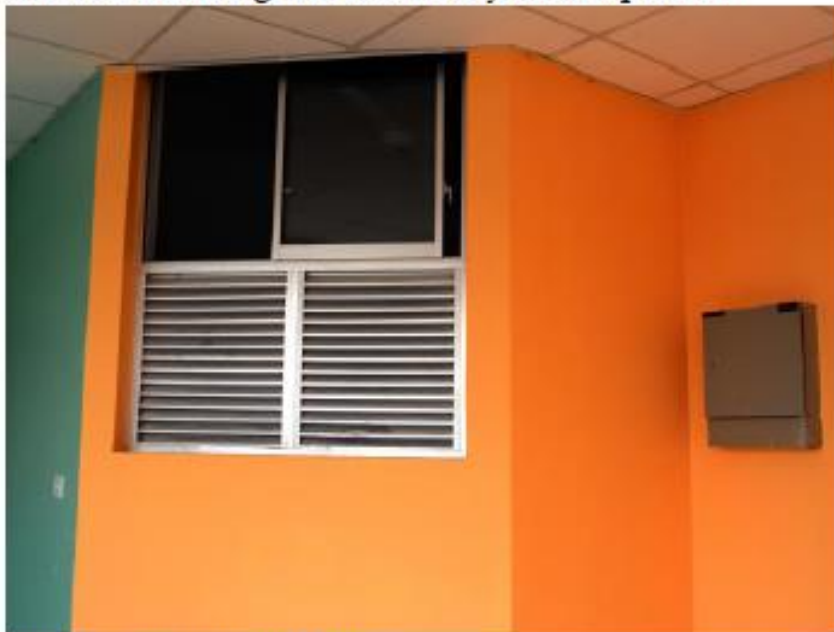
Internal Painting Work
